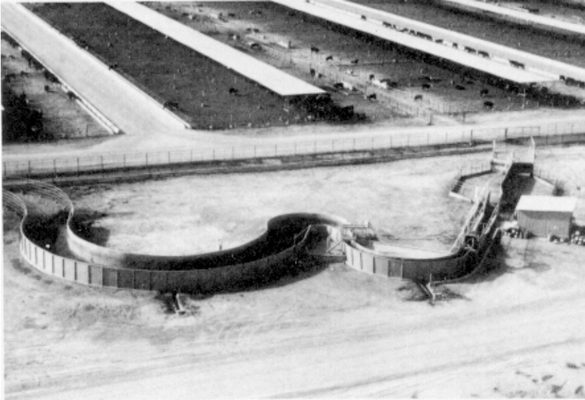
Example of chute using principle of gradual curves suggested in paragraph 16.2.8 (Livestock Markets Association of Canada)
